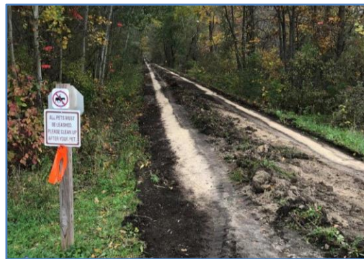
2. A small road grader was used to remove organic material from trail edges
