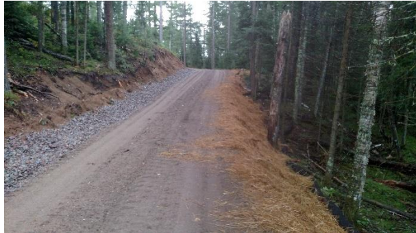
French Drain along Toe of Bench
